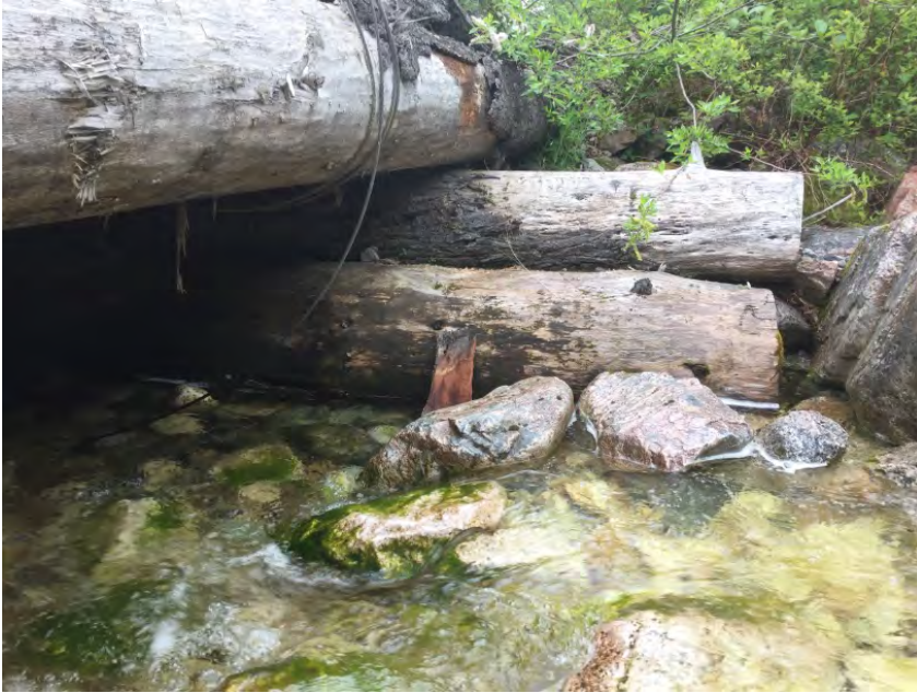
Right Bank Abutment when facing downstream
