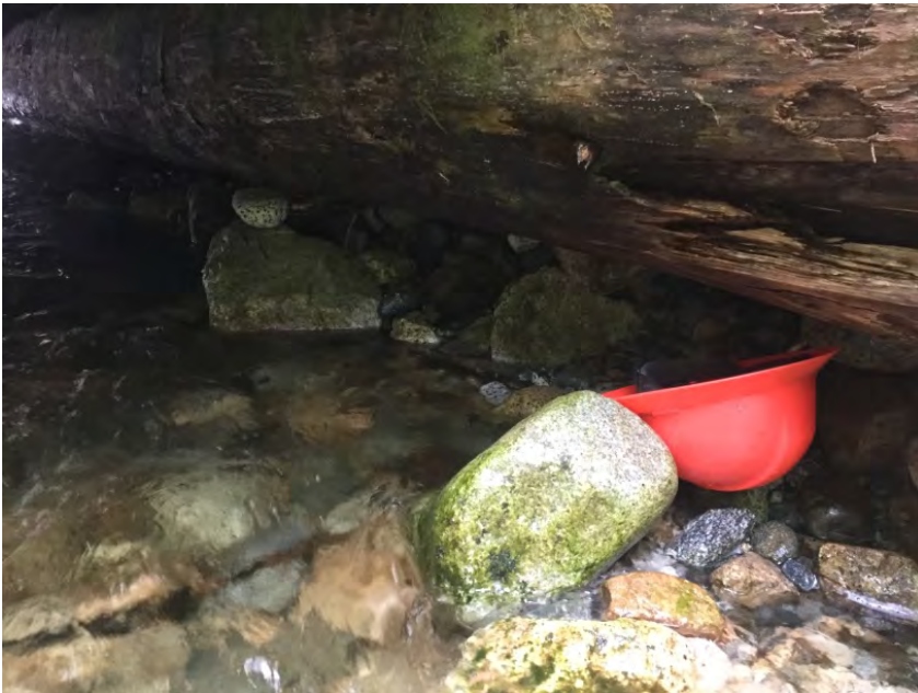
Left Bank Abutment when facing downstream
