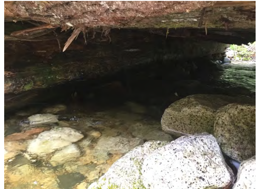
Left Bank Abutment when facing downstream
