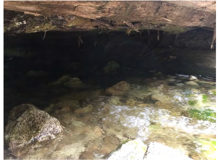
Right Bank Abutment when facing downstream
